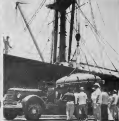
two condensers dwarf the man between them, and at right a condenser head is loaded directly on a truck. na banda di waf. Na centro, e condenser-nan, y na drechi, un condenser head" ta worde descargá ariba truck.
